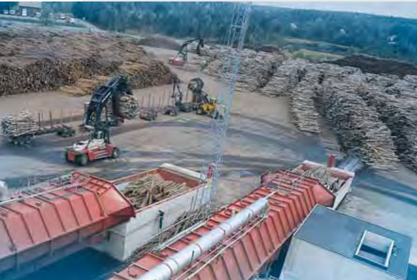
Wood handling, debarking, chip cutting and chip handling
