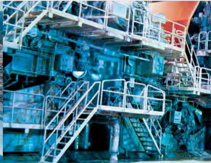
Fiber line, wet end, dry end and coating
