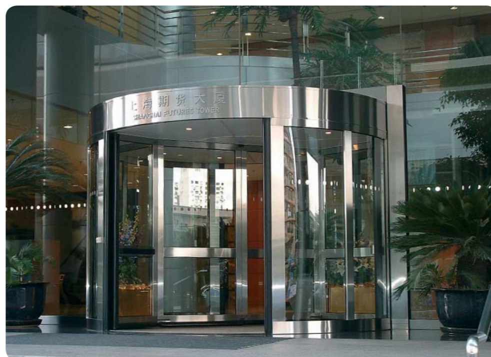
Future Tower – Shanghai, China
