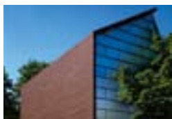
Universidad Stuttgart, Stuttgart, D Rolf Loew, Stuttgart Dangel GmbH, Lenningen TECU® Oxid
