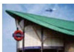
Estación de metro Hounslow West, Londres, GB Michael Watkins (Partner), Londres, (Acanthus, Lawrence and Wrightson Architects) Broderick Structures Ltd., Woking TECU® Patina
