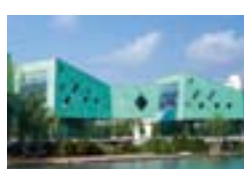
Yefei's Creative Street, Shanghai, VRC Will Alsop Architects, Londres, GB; U/Jiang Architects & Engineers, Shanghai Hanchang Industrial Development Co., Shanghai TECU® Patina, TECU® Oxid, TECU® Bronze
