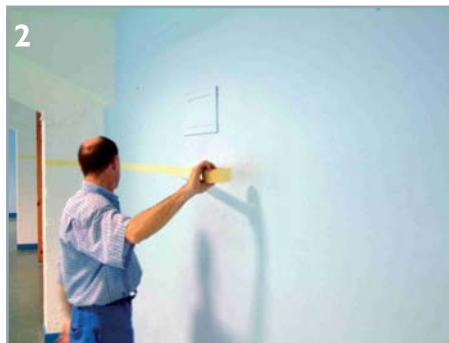
2 Delimitar la zona a acolchar Delimit the zone to quilt Delimitar la zone de travail
