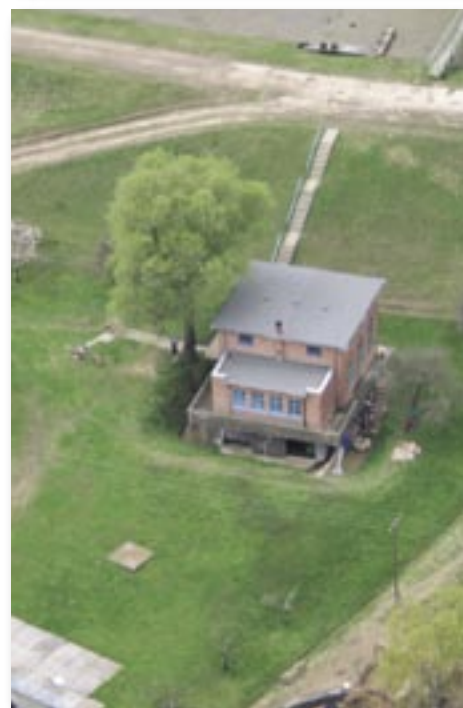
Pump station behind dyke
