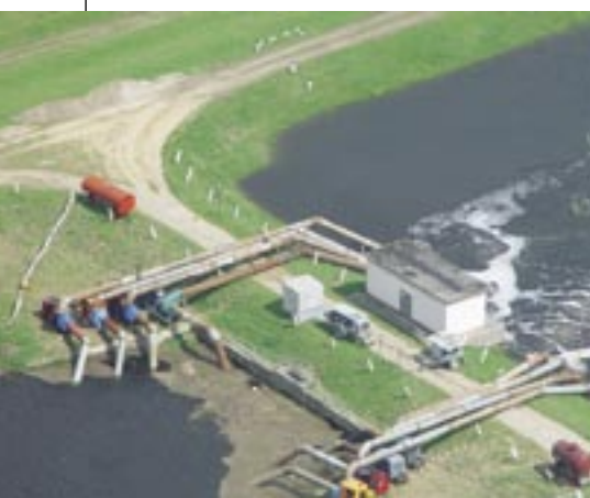
Temporary pump installation at place where flood water meets inland water
