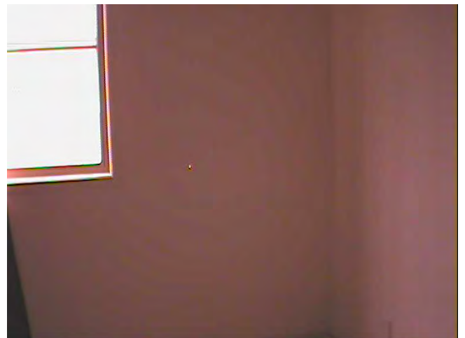
Figure 4b. Visual image shows no signs of termites
