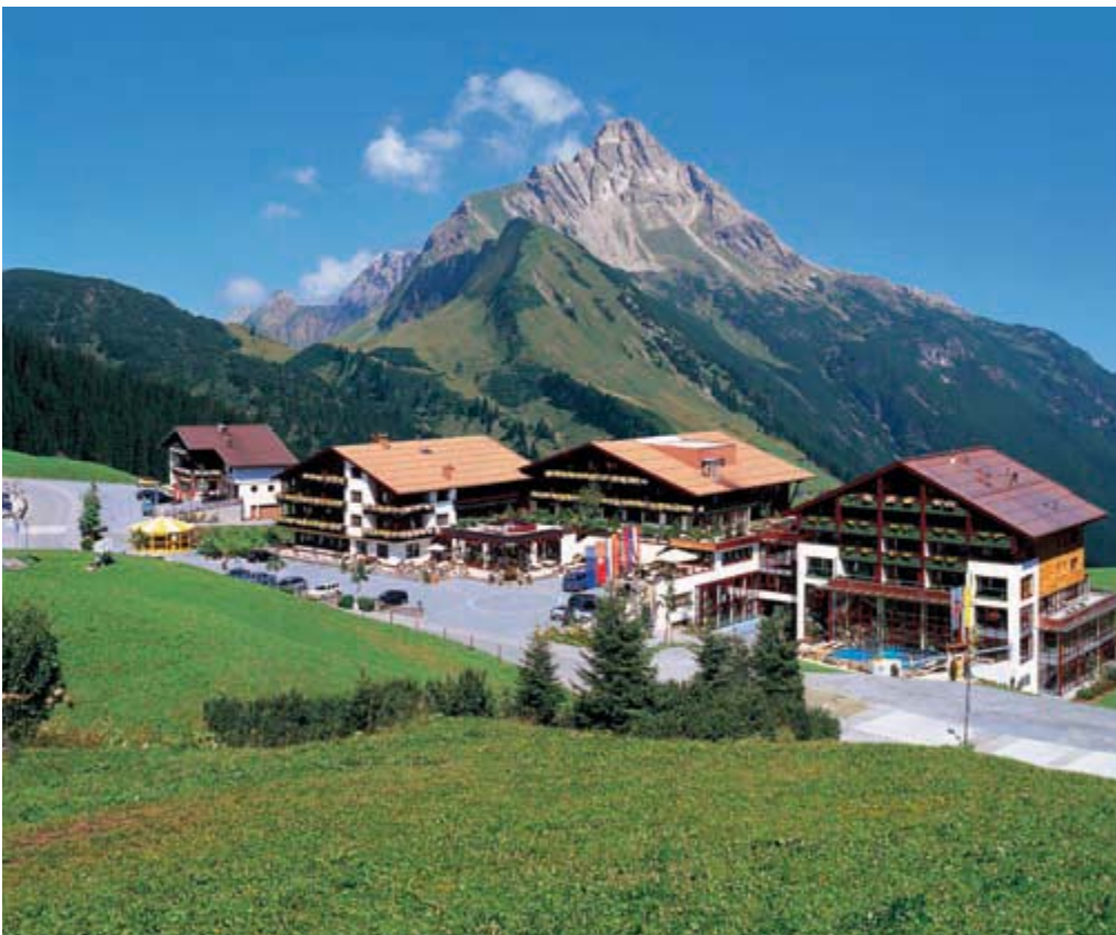
Hotel Wellness Warther Hof, Warth am Arlberg, Austria Arquitectura: Estudio Krissmer & Partner GmbH
