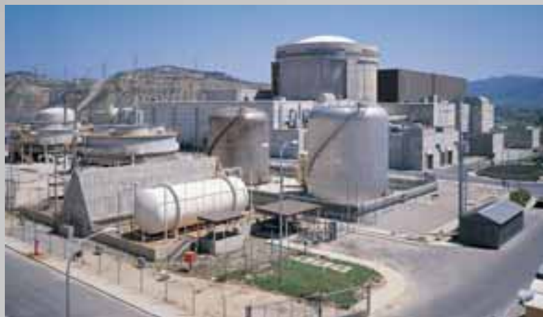
Centrales Nucleares - Nuclear Power Station
