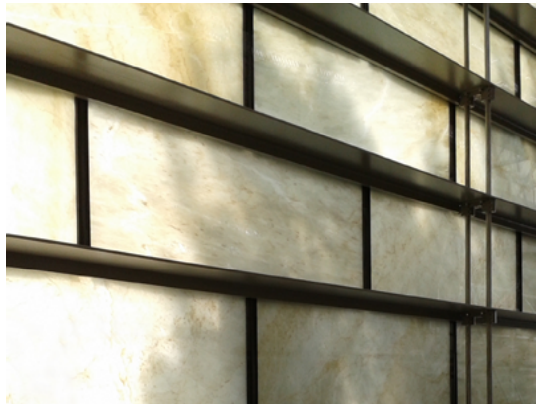
Curtain wall in the Contemporary Art Museum of Nantes (France)'s with Ceptual Rock Skin® (image above).
