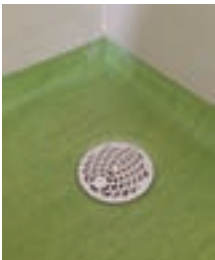
Paviment Vinílic antilliscant Tarkett Optima Multisafe a Hospital de Vic
