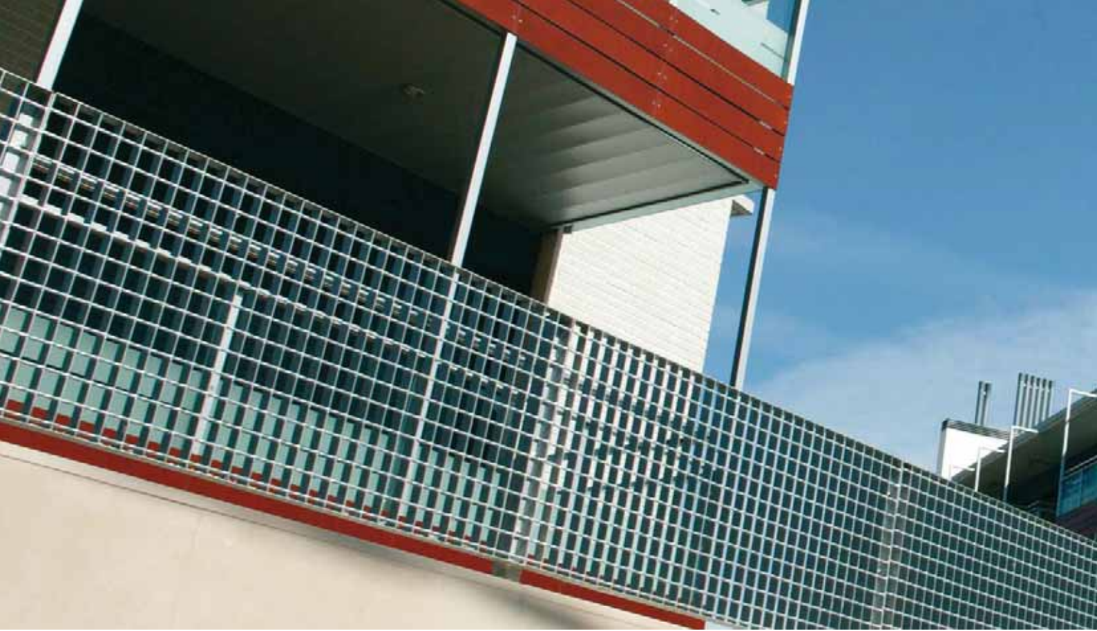
Block of flats in Tiana, Barcelona. Eduard Sabater. Hollow Brick. Ref. White Marble Construction project finalist in the private works category in the Maresme 2004 Triennial Architecture competition
