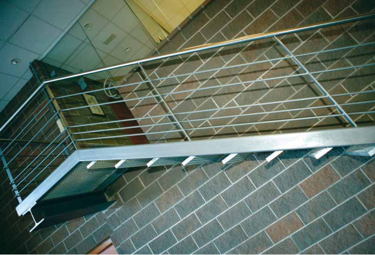
Office in Canovelles, Barcelona. Split face Block. Ref. Sierra / Oficinas en Canovelles, Barcelona. Bloque Split. Ref. Sierra
