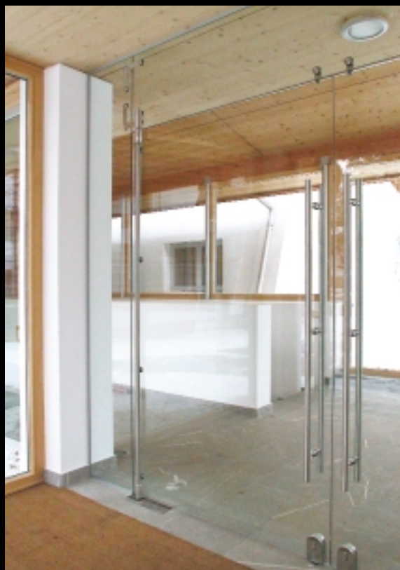
Primary school entrance area, Natz, Italy
