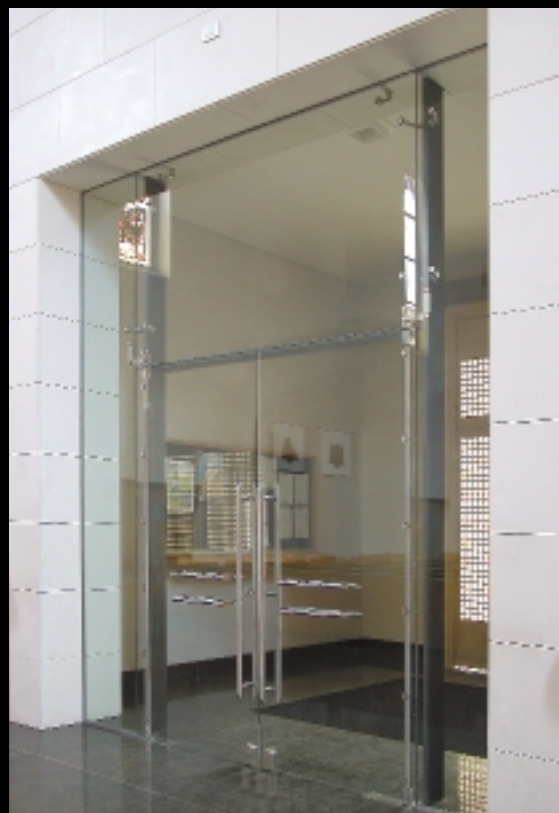
Entrance area of Don-Bosco Church, Bolzano, Italy (with cross formed by MANET pull handles)
